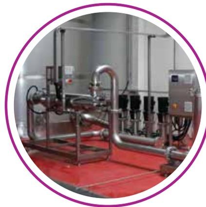
Water which will be disinfected via UV light, must be filtered, purified from hardness and heavy metals such as irons and manganese.
